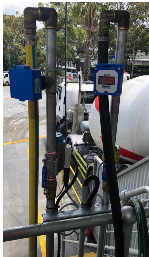
Water Slumpstand at a Premix Concrete Batch Plant MRTU4-GAL25-T2 25mm size flowtube
