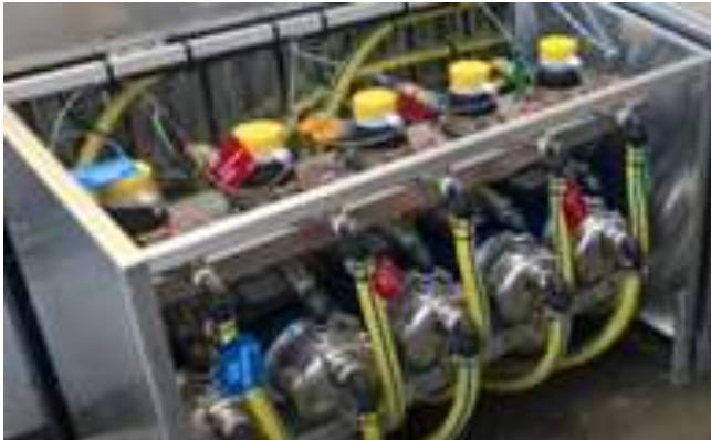
MES20 20mm flowmeters install
