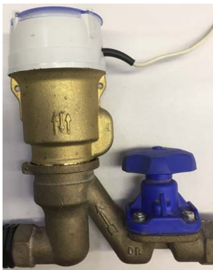
15mm rated (NZ) unit on manifold
