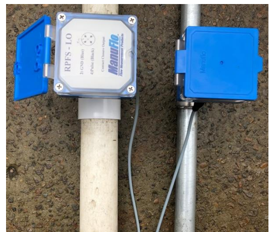
RPFS-LOD installed on a 50mm PVC pressure pipe line and 25mm galvanised steel pipe, using PVC50 and GAL25 adaptors.
